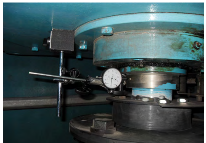
Runout inspection on slip-ring assembly
