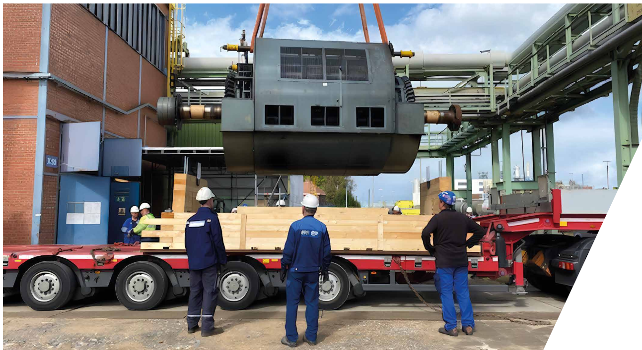
Removal of the damaged generator by our expert staff
